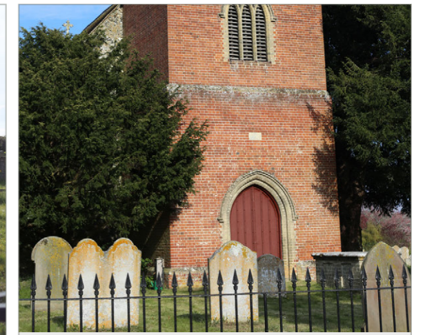
St Andrew's Church on the east of Church Street in Layham to the right of the viewpoint.
