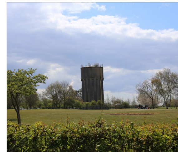
To the south-east of the viewpoint, Raydon water tower is a distinctive skyline feature.
